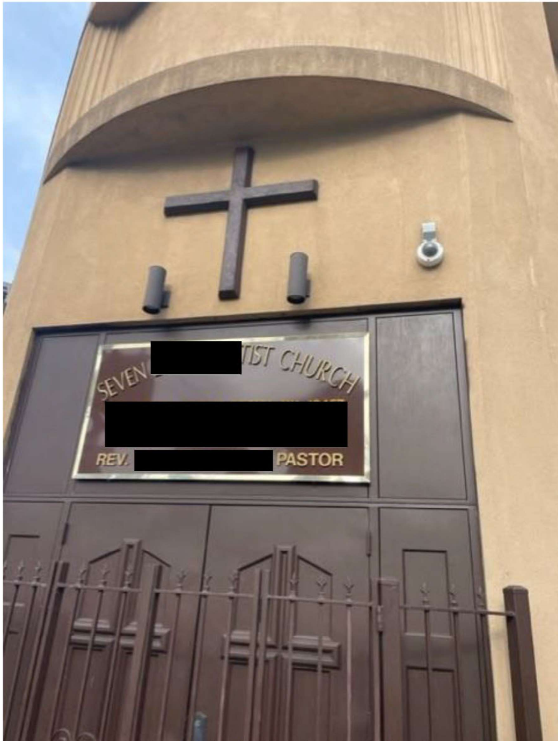
Camera observed on Seven Adventist Church, which sits on the northwest corner facing intersection.
