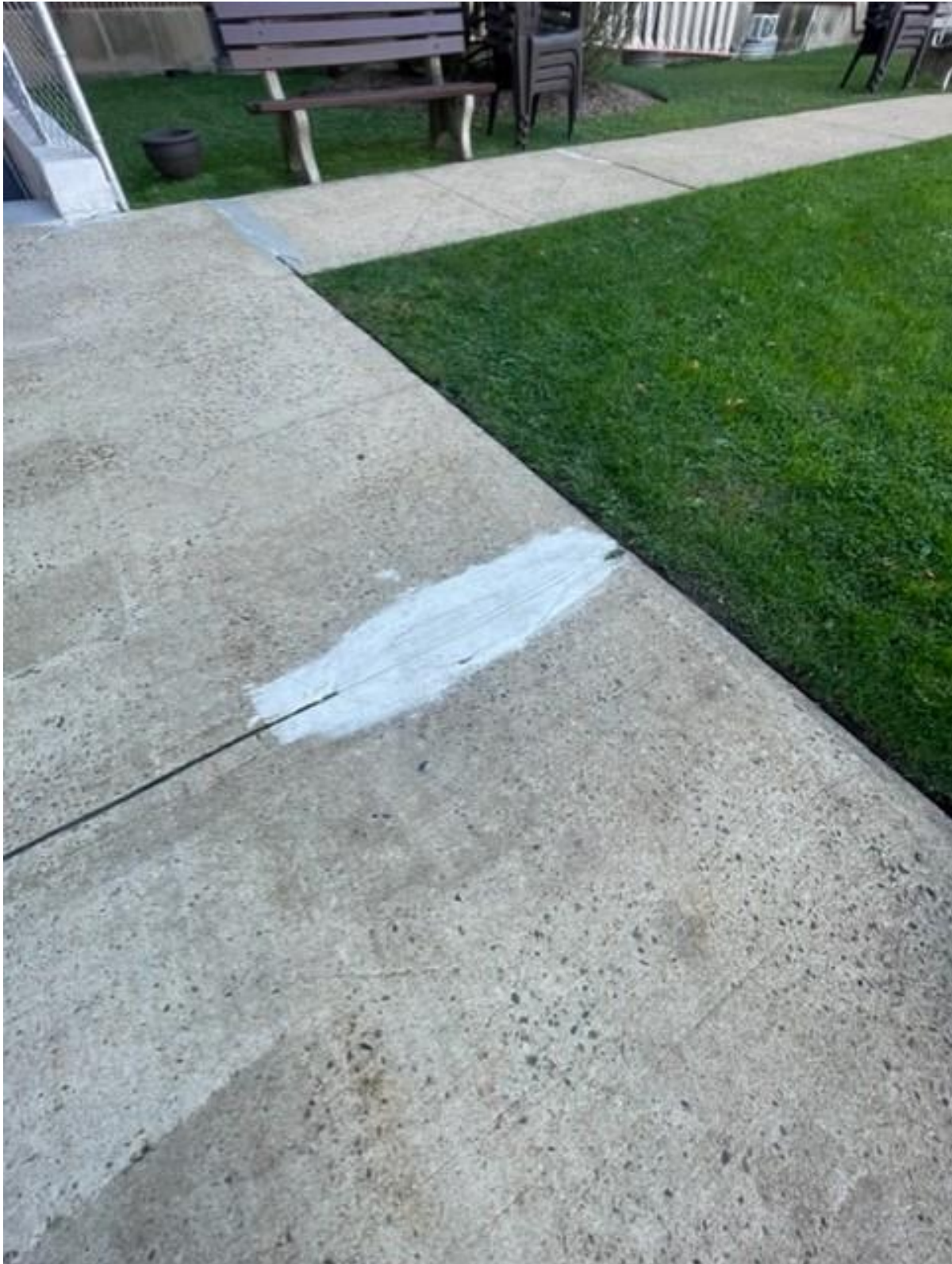
Closeup of repair to walkway.
