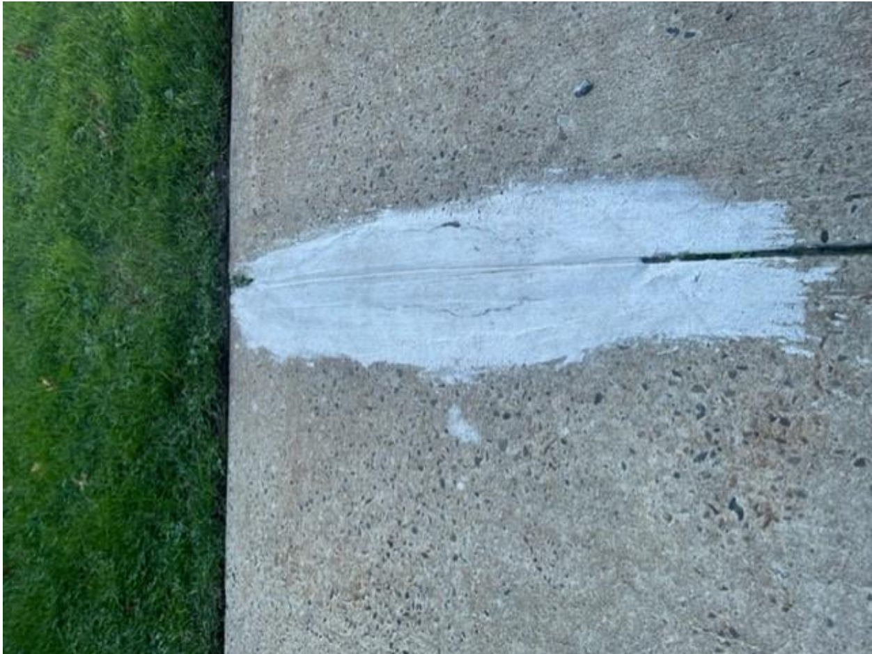
Closeup of repair made to walkway.
